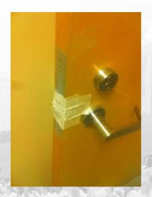
Door propping is unacceptable because it reduces the fire rating of the room in the case of a fire, allowing smoke and/or fire to spread.
